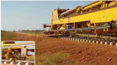
Harsco Track Laying Machine with integral clip application module
