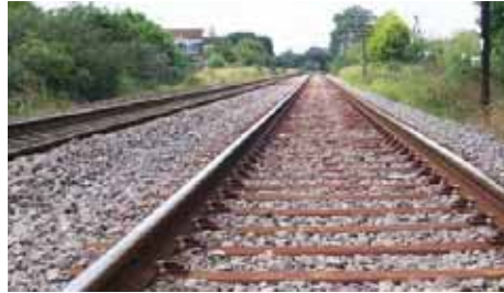
PANDROL FASTCLIP steel sleeper installation
