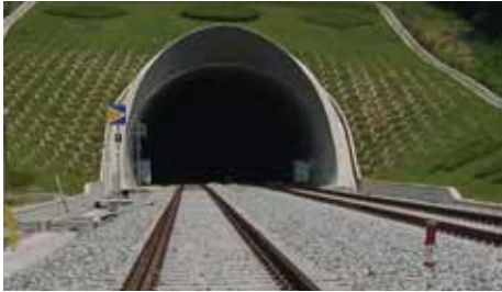
PANDROL FASTCLIP concrete sleeper installation
